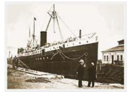
The Colorado in the drydock at Hunter's Point in San Francisco
